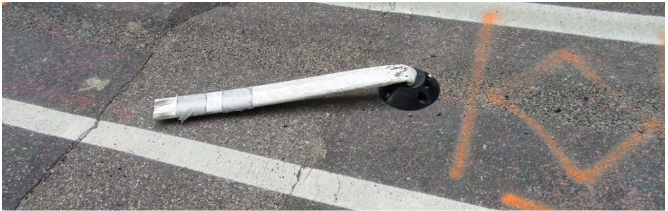
Figure 58: Bollard not maintained
