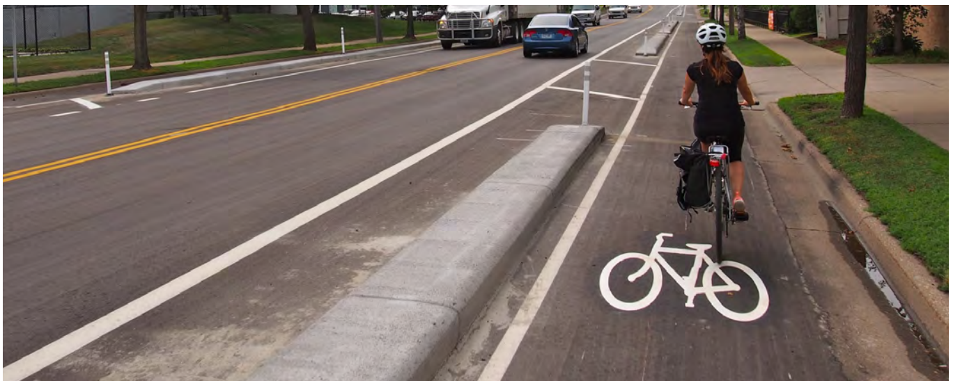
Figure 60: Curb separated bike lane prevents temporary parking in lane
