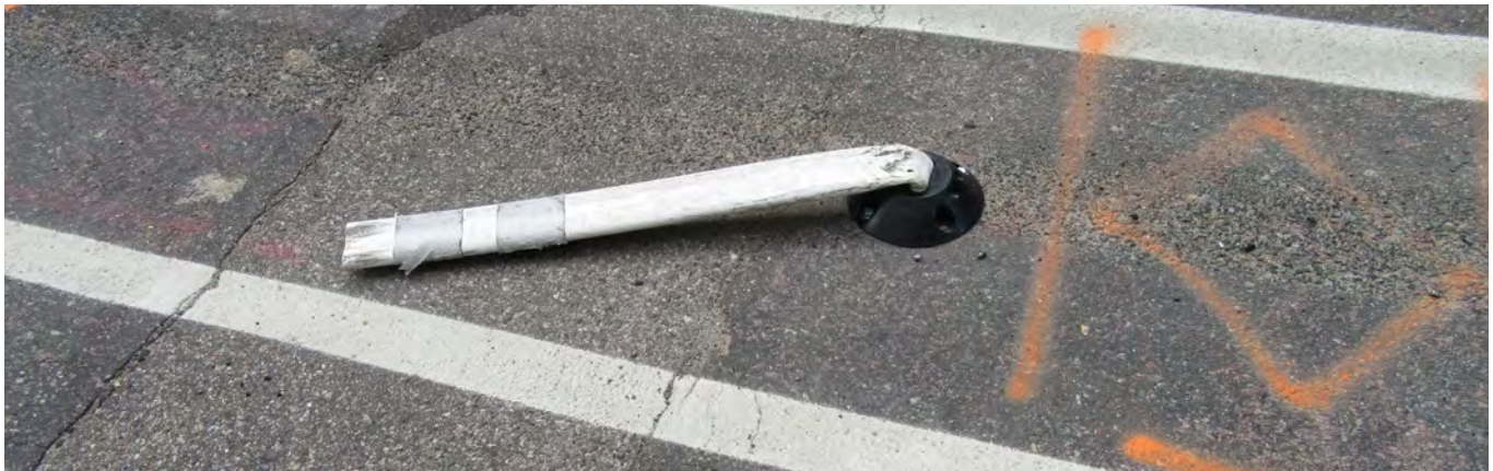
Figure 58: Bollard not maintained
