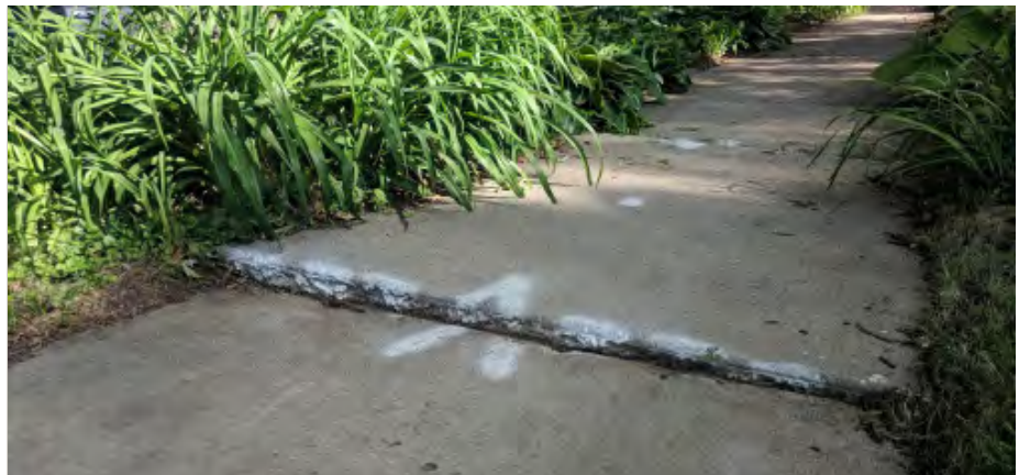
Figure 38: Sidewalk gap (on left) filled with the construction of new sidewalk (on right)
