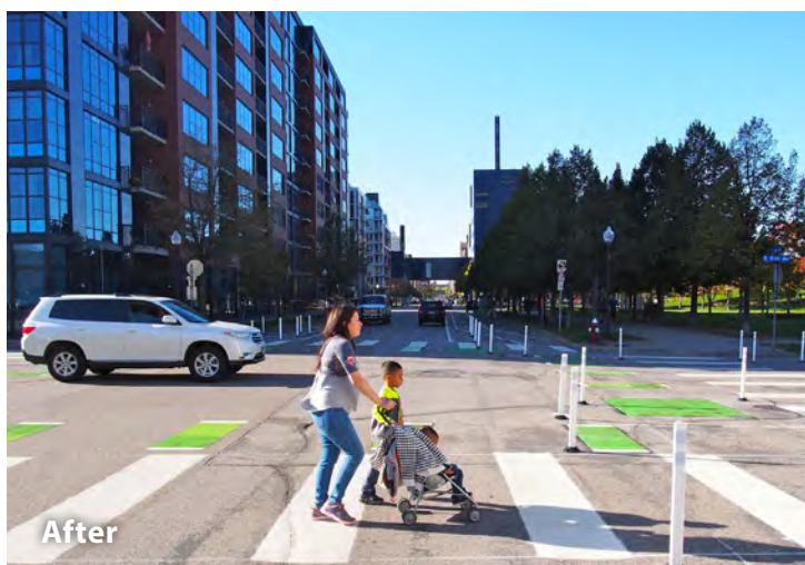
Figure 25: Paint and bollards improve conditions for people walking and bicycling; 11th Avenue and 2nd Street S
