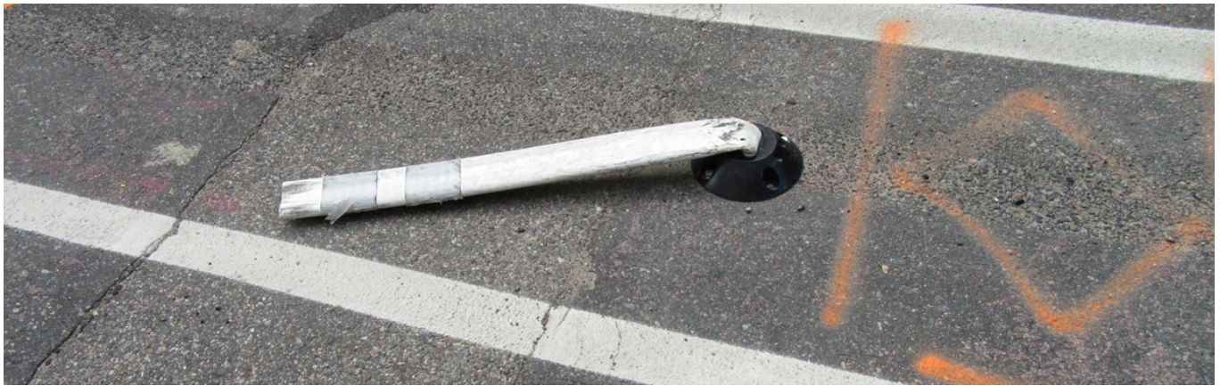
Figure 60: Bollard not maintained
