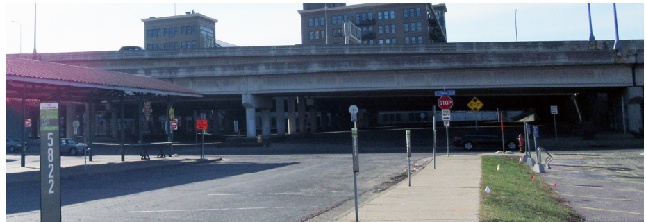
Figure 41: New 5th Street pedestrian bridge over I-35W
