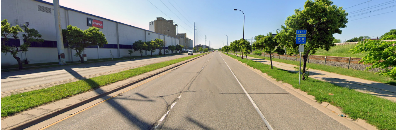
Figure 11: Minnesota Department of Transportation state highway within Minneapolis
