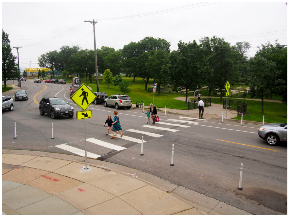
Figure 129: Reconfiguring space on W 15th Street near Loring Park
