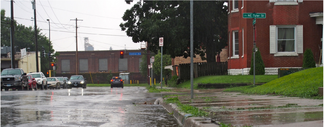
Figure 156: Incorporating stormwater infrastructure on street projects will help with localized flooding issues
