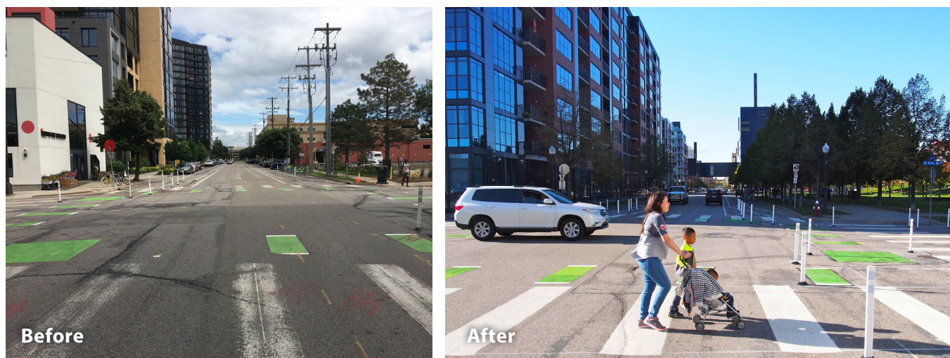
Figure 26: Paint and bollards improve conditions for people walking and bicycling; 11th Avenue and 2nd Street S
