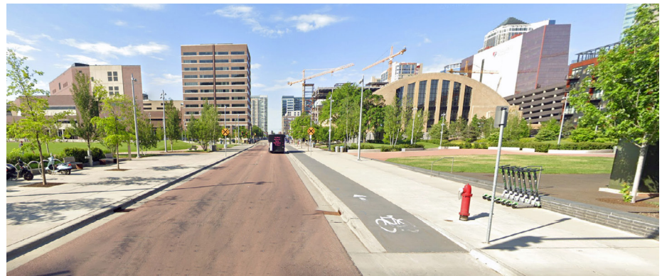
Figure 43: Protected bikeway and enhanced pedestrian realm near The Commons Park
