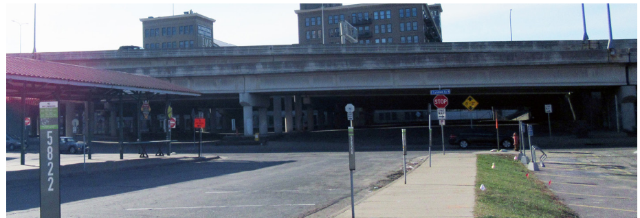
Figure 41: New 5th Street pedestrian bridge over I-35W
