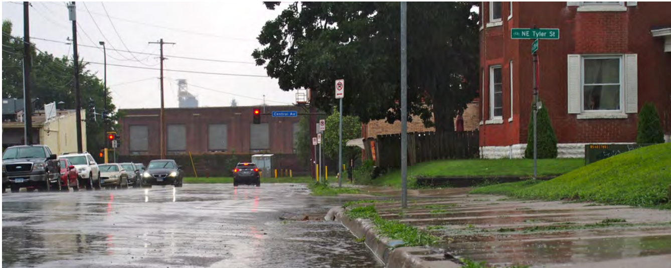
Figure 156: Incorporating stormwater infrastructure on street projects will help with localized flooding issues
