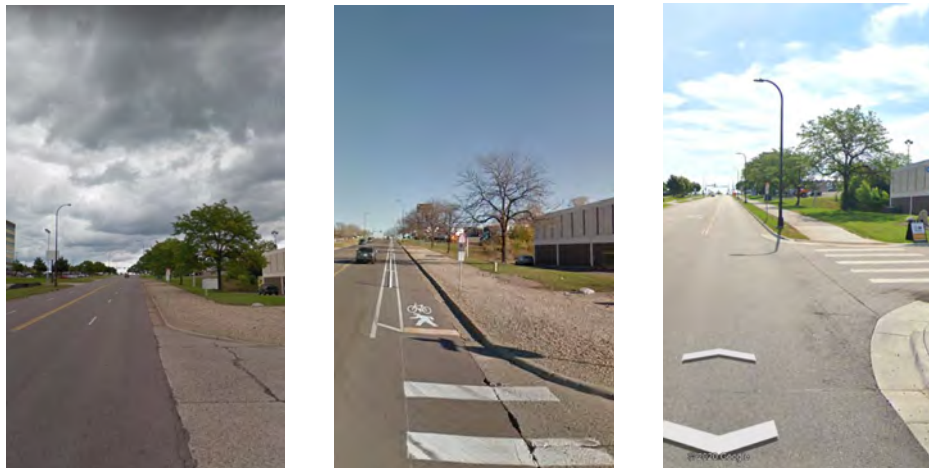
1 Figure 39: Sidewalk gap (left), interim pedestrian facilities (middle), and new sidewalk (right)
