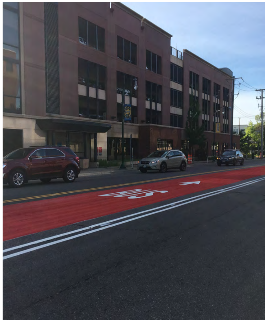
Figure 138: Bus only lane on Chicago Avenue, prioritizes transit travel
