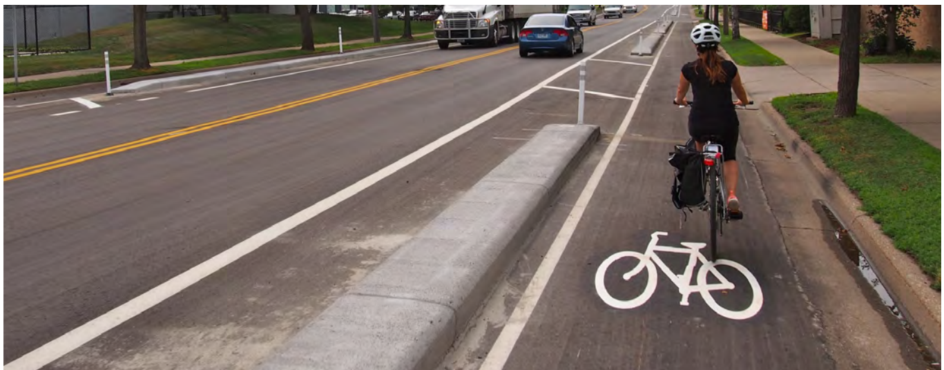
Figure 62: Curb separated bike lane prevents temporary parking in lane
