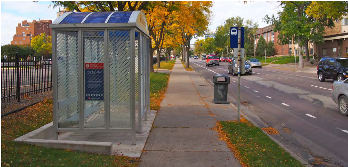
Figure 88: Well maintained transit stop
