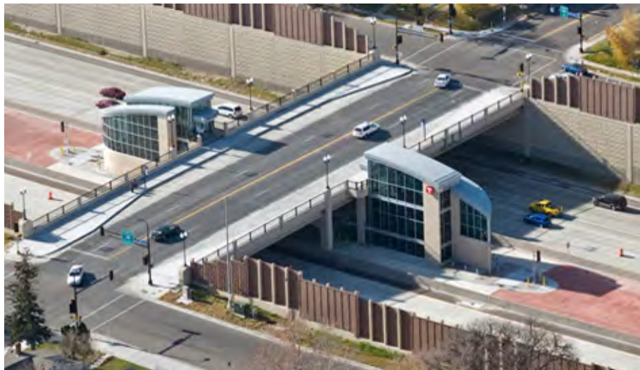
Figure 80: Transit infrastructure on bridge at 46th St S over Interstate 35W
