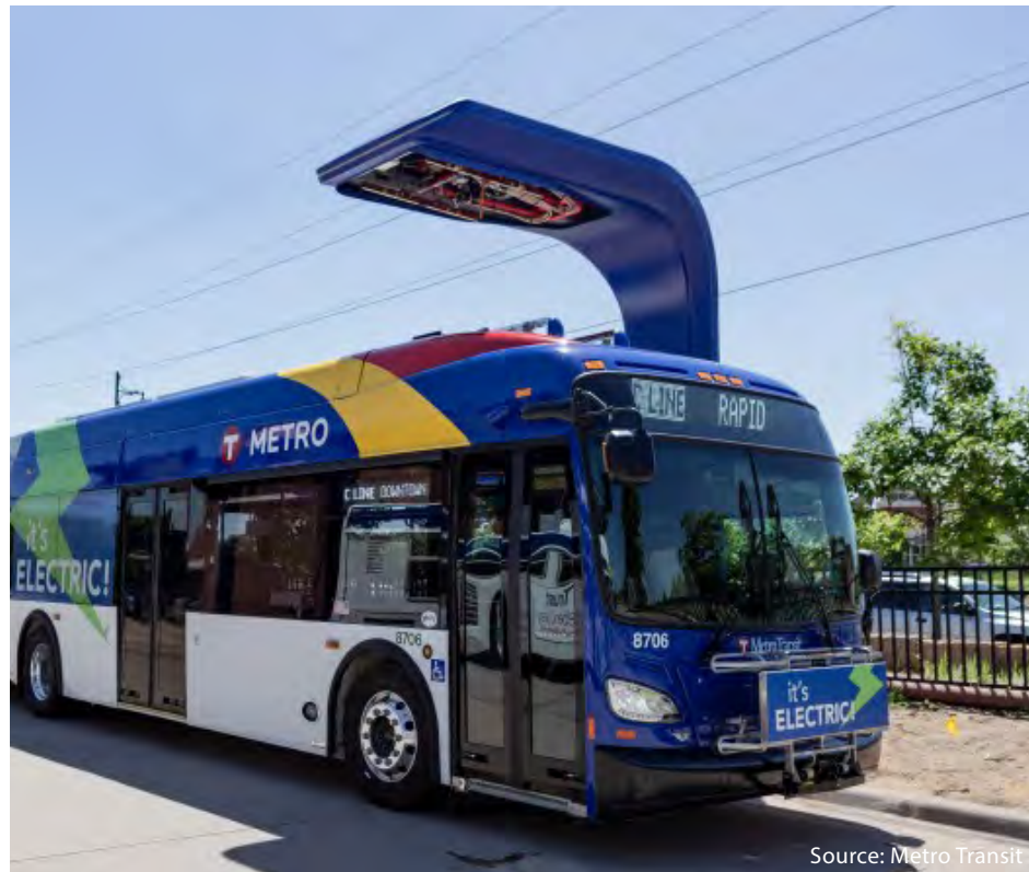
Figure 103: Transit electric charging station – C Line
