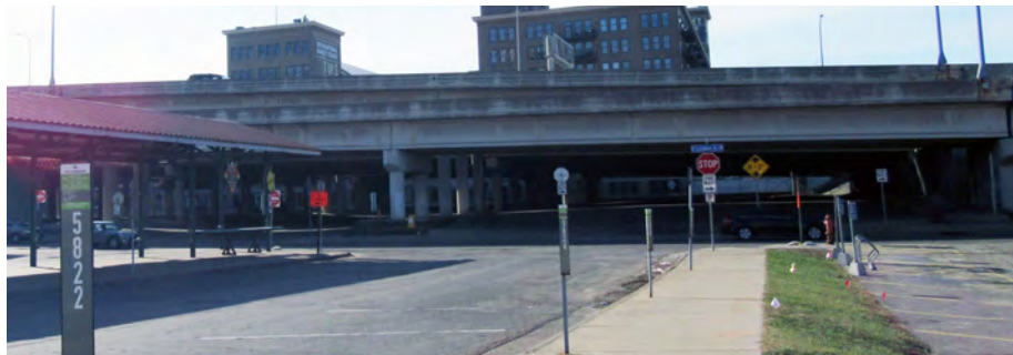
Figure 41: New 5th Street pedestrian bridge over I-35W
